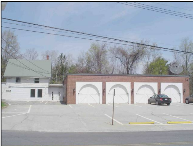
Bedford Cable Television Building
