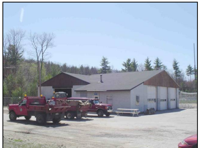
Bedford Park Building
