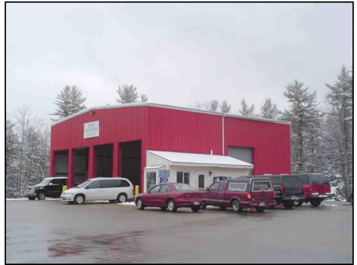
Bedford Transfer Station
