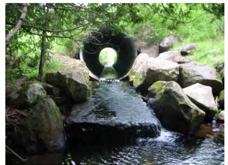
Undersized, perched culvert that has limited flood capacity, cannot pass sediment and large wood, during a flood, and has limited aquatic organism passage.
