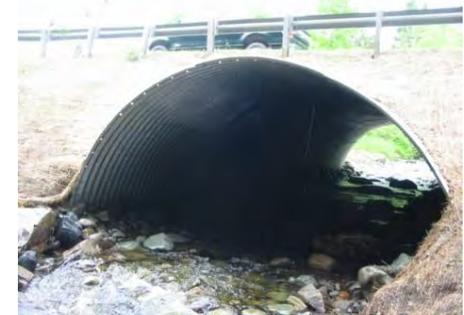
Flood resilient replacement culvert that can pass sediment and large wood during floods, and has good aquatic organism passage.
